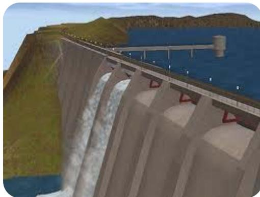
**Introduction** It is a barrier that impounds water or underground streams. It has a section called spillway which is designed to pass water from the upstream side of a dam.
